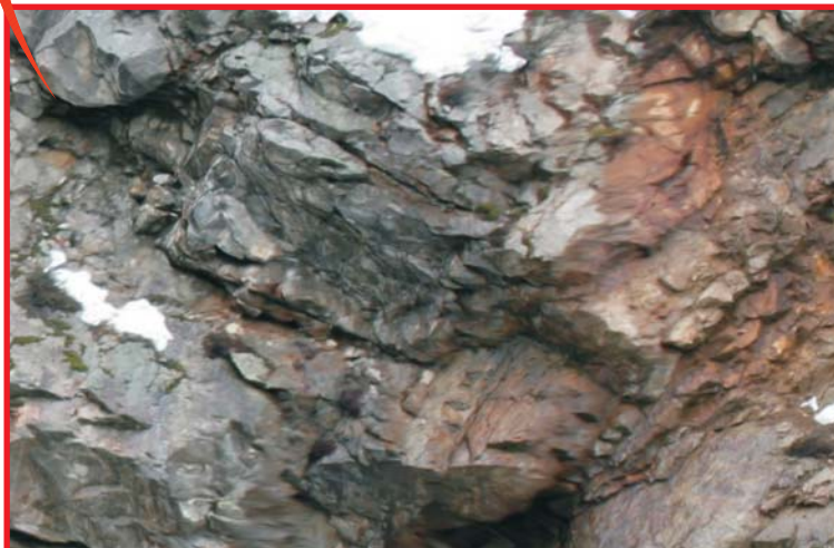
Highway cut - close-up of undercut potential failure block
